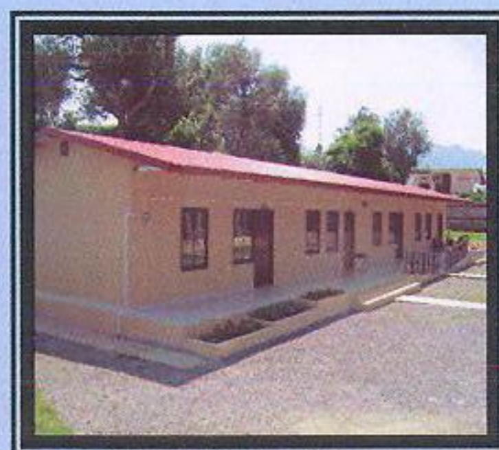
Completed steel structure
